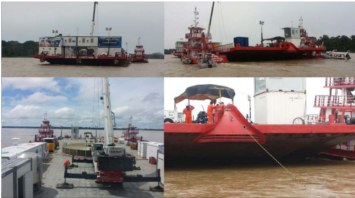
Figure 73: Cable-laying between Coari and Tefé on the Solimões: photos of the equipment used in 2016 (Images from http://www.amazoniaconectada.eb.mil.br/eng/ ) Above: prow and stern of cable laying barge and tugboats; Below left: deck view with one of the reels of cable; Below right: paying out the cable from the stern
